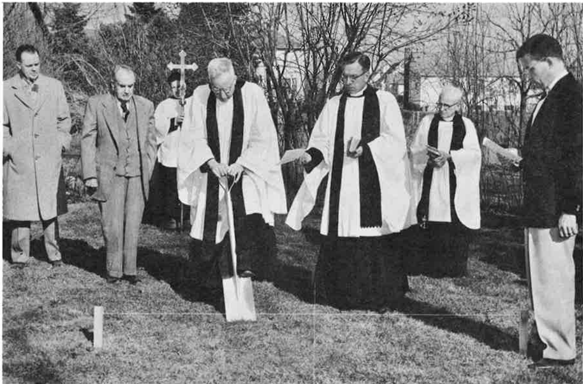
Sod Turning for New Church
